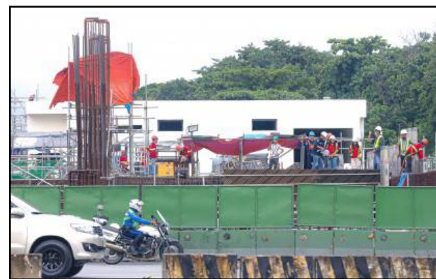
IN PROGRESS. Construction personnel work on the Quezon Memorial Circle Station of the Metro Rail Transit Line 7 (MRT-7) on August 10, 2024. Transportation Secretary Vince Dizon on Thursday (June 12, 2025) assured that the MRT-7 will begin operation by 2027, before the end of President Ferdinand R. Marcos Jr.'s term. (PNA photo by Robert Oswald P. Alfiler)
