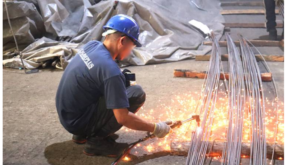
Destruction of Re-rolled bars in Cavite Steel Mill
