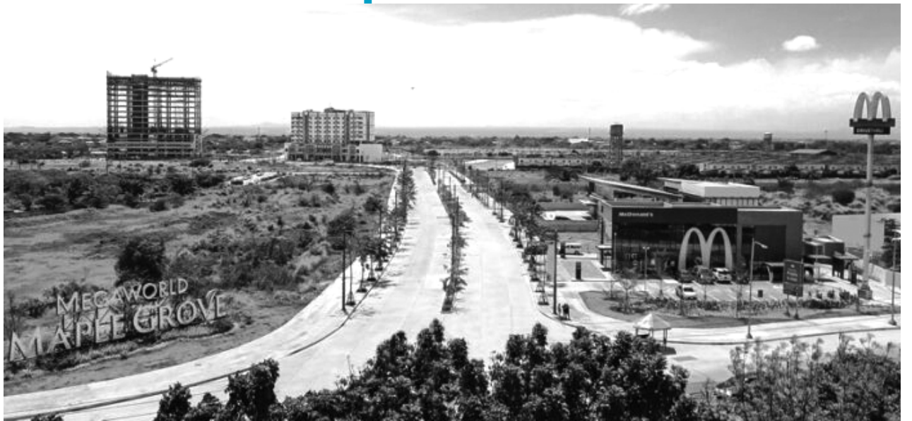
Megaworld's 140-hectare Maple Grove township in General Trias is fast taking shape as Cavite's central business district.
